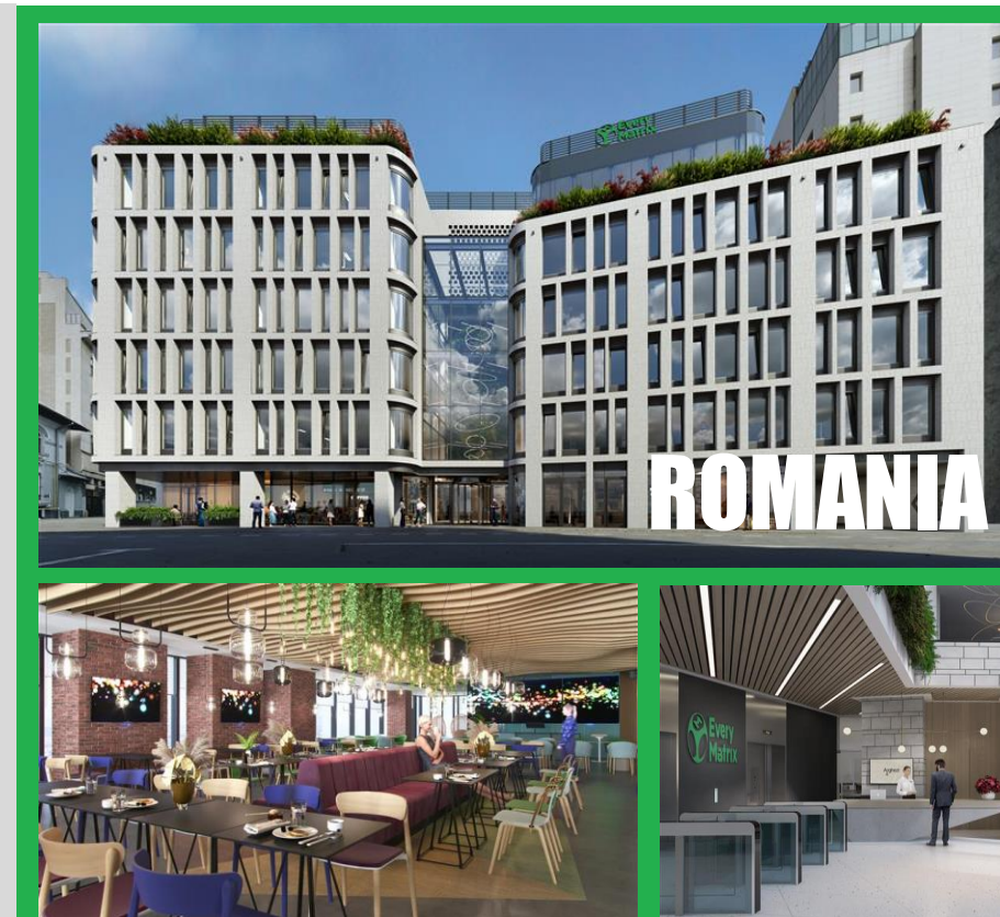
New Bucharest office under construction
